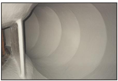
The Cerami-Flex system was selected for this application. A total of 508kg of Cerami-Tech EG were first trowel applied and then a stiff bristled angled paint brush was used to smooth out the high spots and uneven areas. A thickness of 750 microns was achieved.
