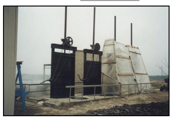
The surfaces were first of all grit blasted to remove all rust and poorly adhered coatings.
